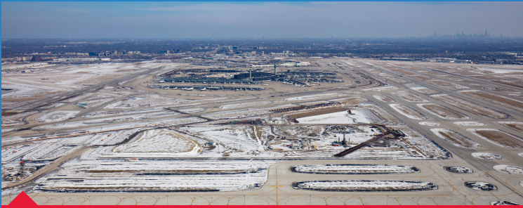
CDA, American Airlines, and United Airlines unveiled a new Central Deicing Facility (CDF) at O'Hare in February. The size of 17 football fields and the largest facility of its kind in the U.S., the CDF will help reduce gate delays during winter weather.
